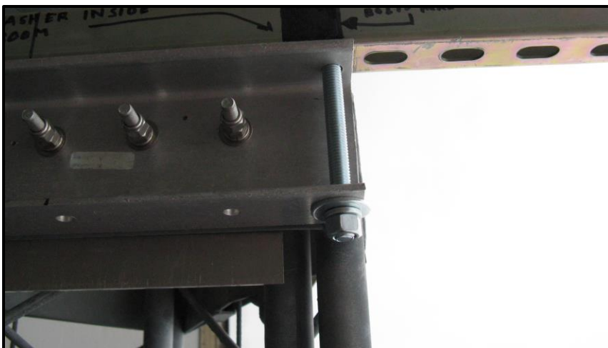
Figure 19 - Washer, lock washer and nut in place
