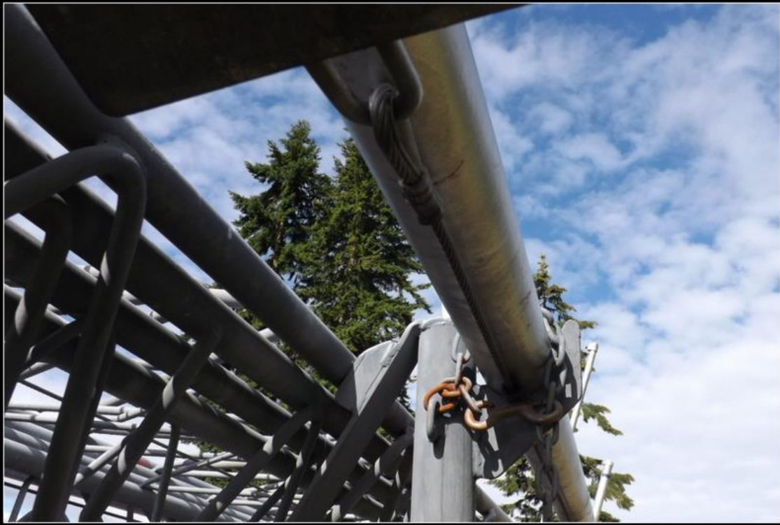
Figure 6 - Opposite Safety Retainer Chain
