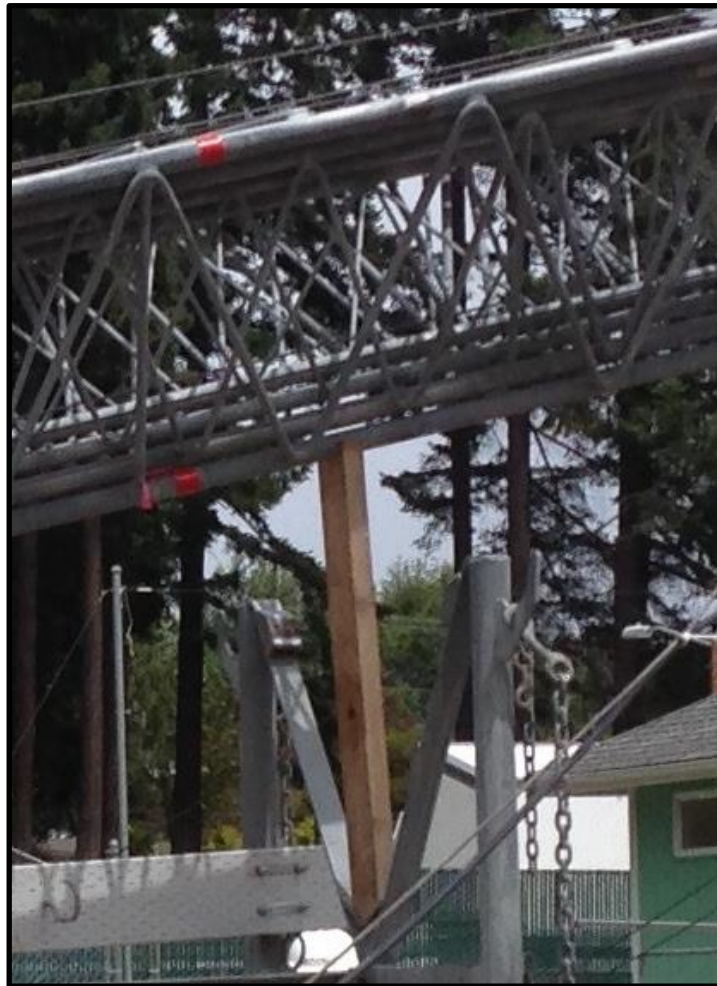
Figure 20 - 2x4 Safety Support
