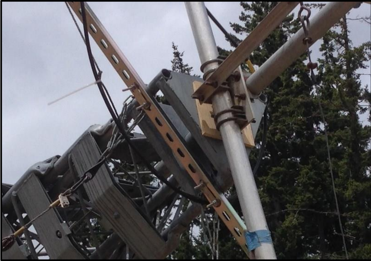
Figure 21 - Detail of Mast Mount – NOTE - this is the old crossbar installation. See Phase 3 for new crossbar mount.
